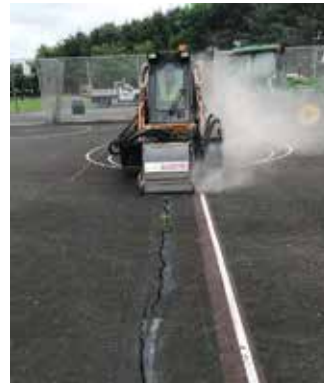
Windlestrae Park - Rose Twig – Repairs were made to cracks on one of the basketball courts to ensure safe playing and the same type of repairs will be made on the second court this spring/summer.
