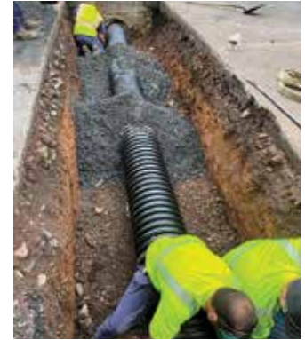
Replacing a deteriorated corrugated metal storm sewer pipe with a more durable polyethylene pipe across Grays Lane.
