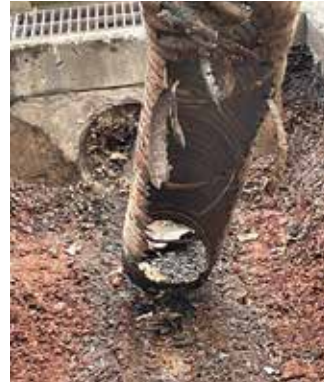
Replacing a deteriorated corrugated metal storm sewer pipe with a more durable polyethylene pipe across Grays Lane.
