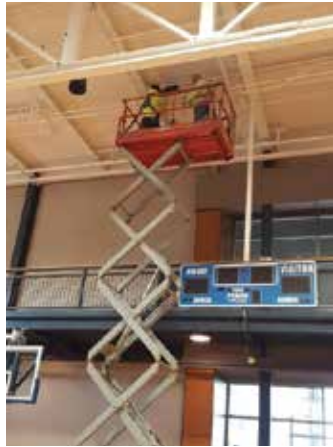
Repairing the lighting in the gym of the CRC building.
