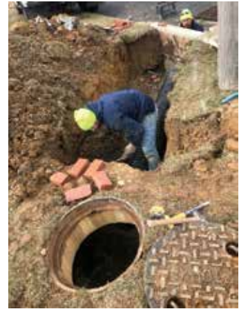
Replacing a deteriorated storm sewer pipe at Stump Rd. & Commerce Dr.
