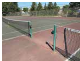
Crack repairs and new color coating and striping on the tennis courts
