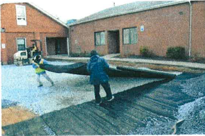
Installation of woven monofilament geotextile. (TOP LEFT). Compaction of Stone (TOP RIGHT). Final Bedding layer (BOTTOM LEFT). Installation of mats and individual blocks (BOTTOM RIGHT).
