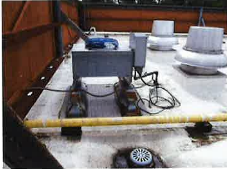
Computer Room Air Conditioner Condenser Unit
