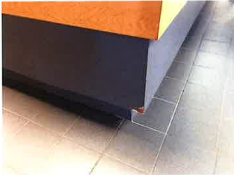
Damaged millwork
