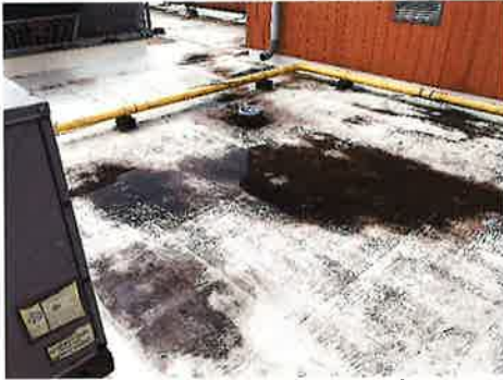
Evidence to ponding on roof
