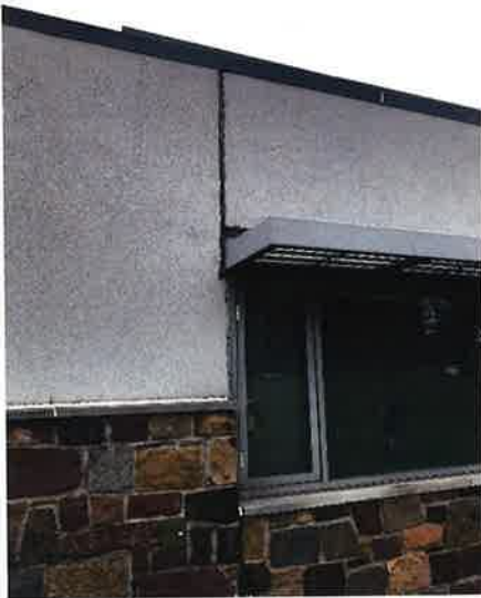
Repairs to plaster control joint
