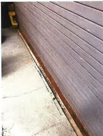
Overhead door sill oxidation
