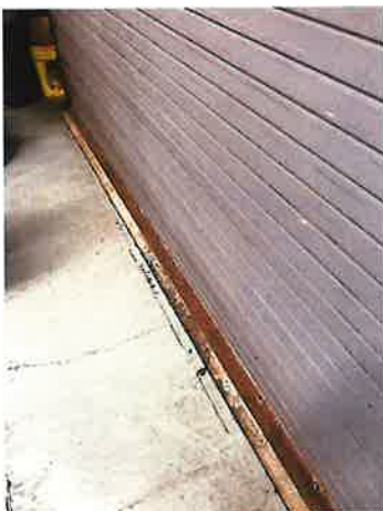
Corrosion at Door Sill
