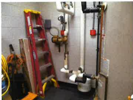
Domestic Hot Water Heater And Recirculation Pump
