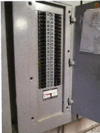
Typical Electrical Panel – Limited Capacity
