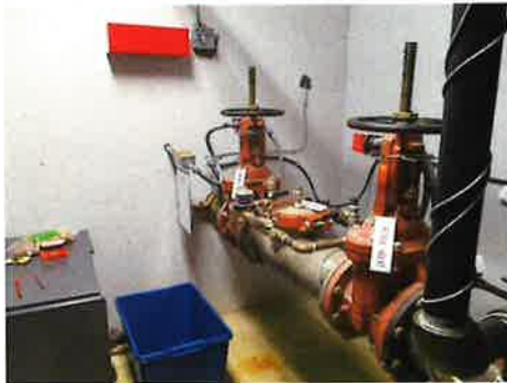
Fire Protection Water Service Entrance (Domestic Service Behind)
