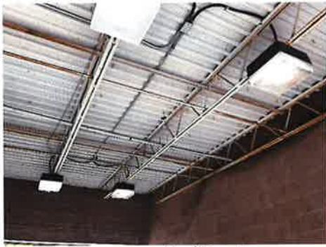
Corrosion at Roof Framing
