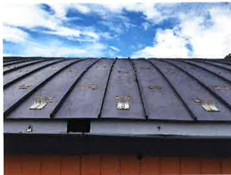
Damaged gutter and missing roof guards
