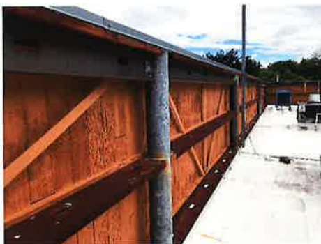
Oxidation on roof screen framing
