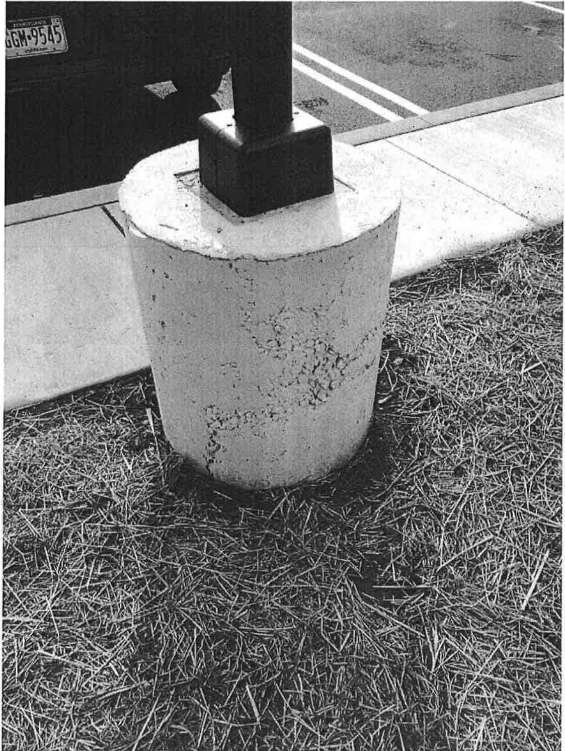
Foundation Observation Photo No. 3
