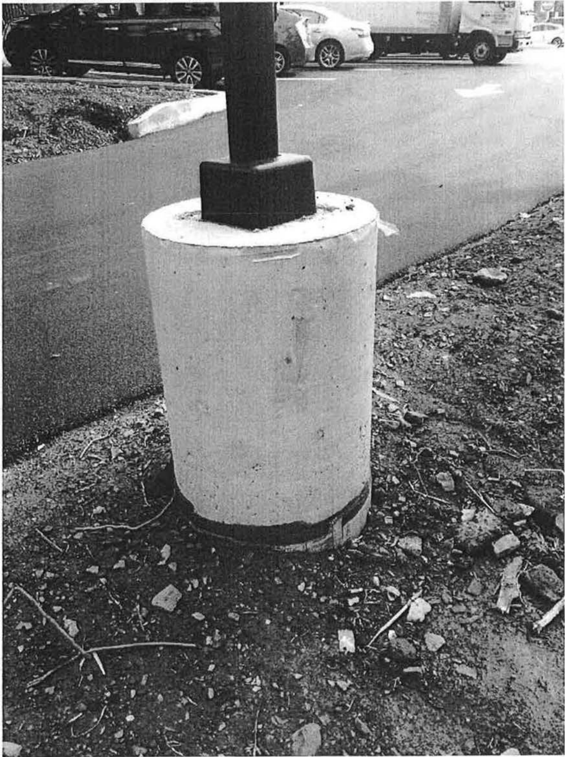
Foundation Observation Photo No. 1
