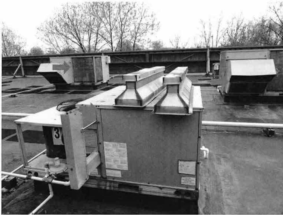
Photo 7 - Roof Area A -View of the rooftop equipment (red arrows) inside the screen wall near the roof hatch and above the insulated fully adhered EPDM roof system
