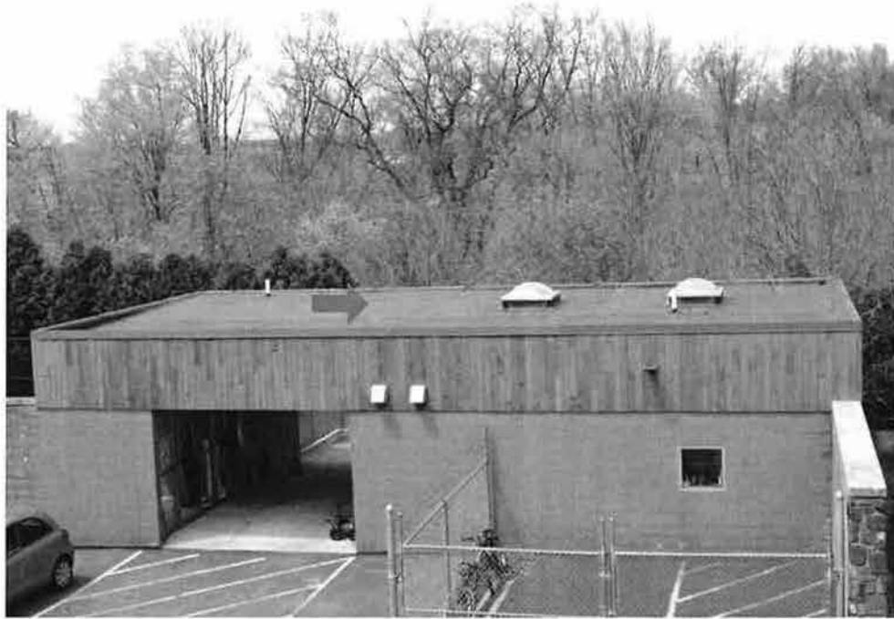
Photo 27 - Roof Area E - View of the insulated fully adhered EPDM roof system (red arrow) on the Dog Kennel Building.
