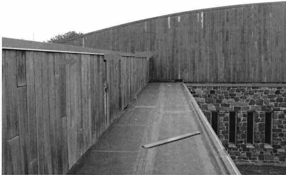
Photo 23 - Roof Area D - View of the screen wall (red arrow) above the insulated fully adhered EPDM roof system.
