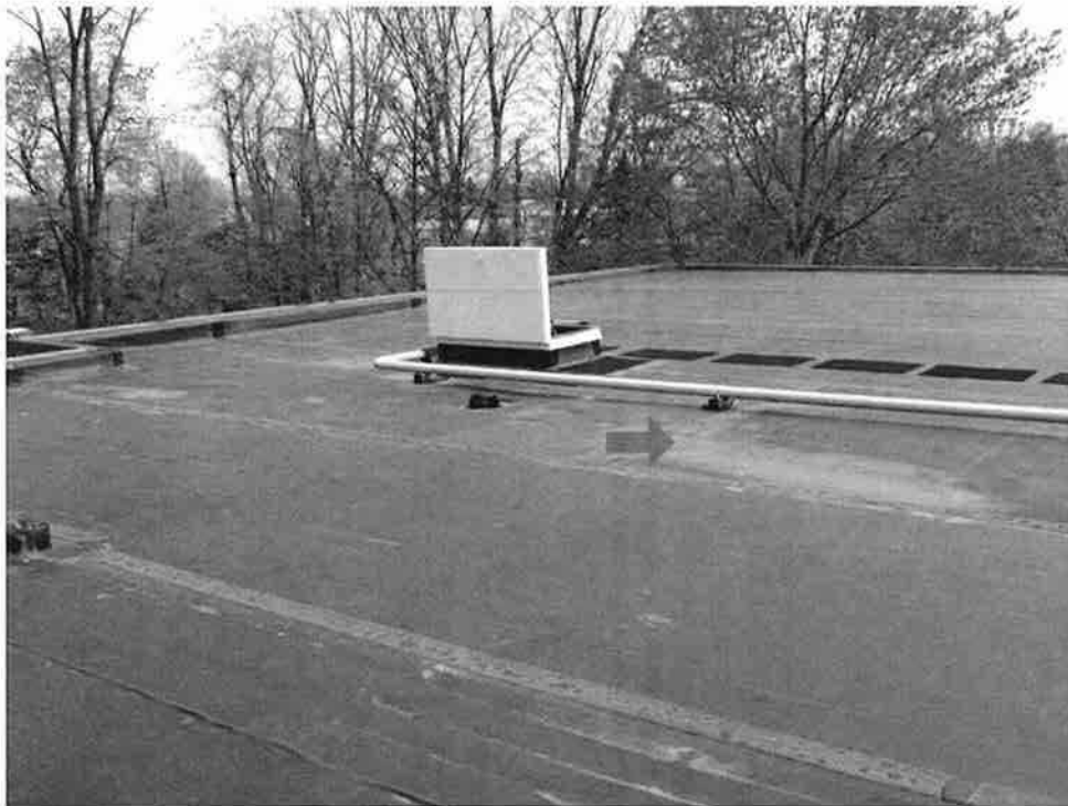
Photo 4 - Roof Area A -View of areas of roof where water ponds (red arrow) on the insulated fully adhered EPDM roof system
