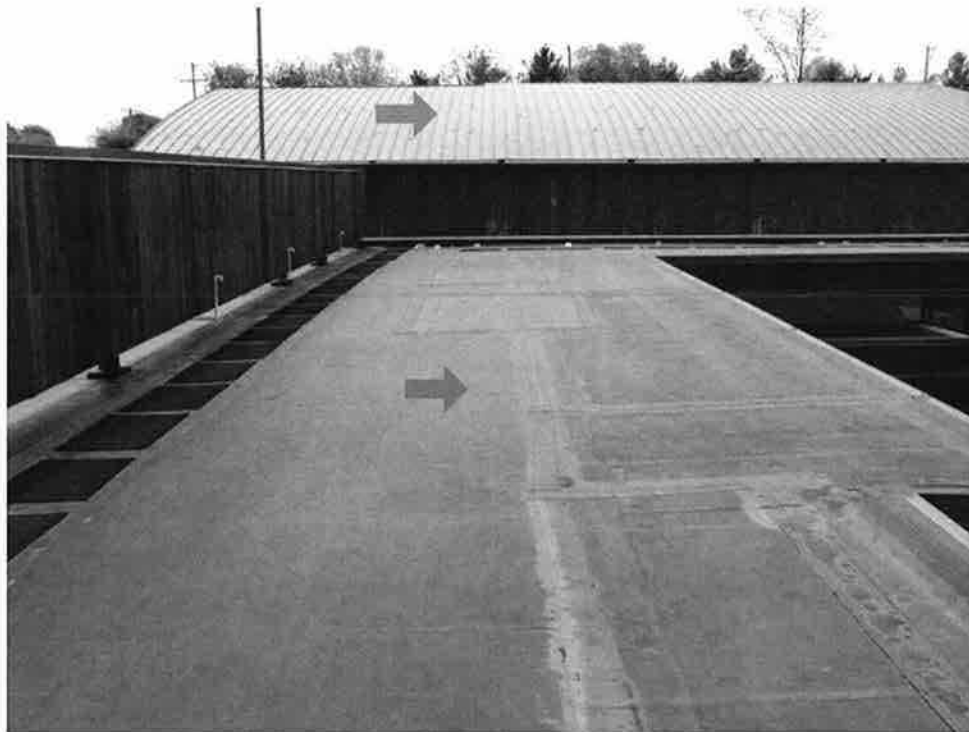
Photo 6 - Roof Area A -View of areas of the insulated fully adhered EPDM roof system (red arrow) in front of the Upper Metal Roof (green arrow)
