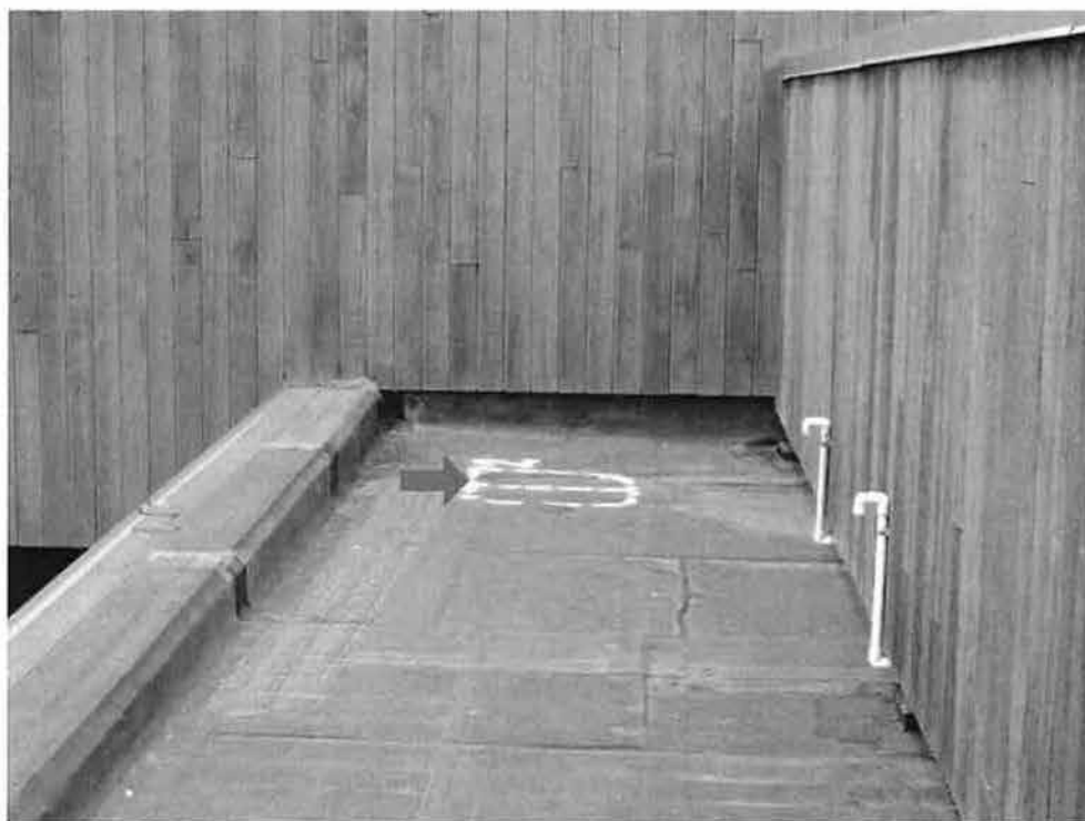
Photo 13 - Roof Area A -View of the location of water trapped in the insulated fully adhered EPDM roof system (red arrow) in Anomaly 2 adjacent to Roof Area B.
