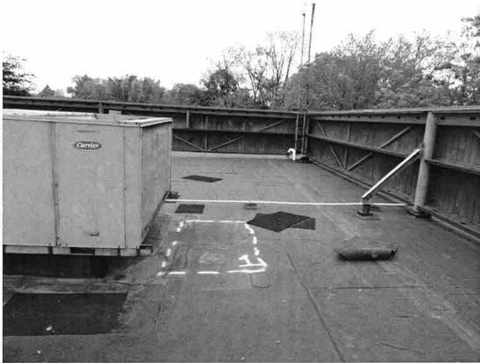
Photo 11 - Roof Area A -View of the location of water trapped in the insulated fully adhered EPDM roof system (red arrow.) in Anomaly 1
