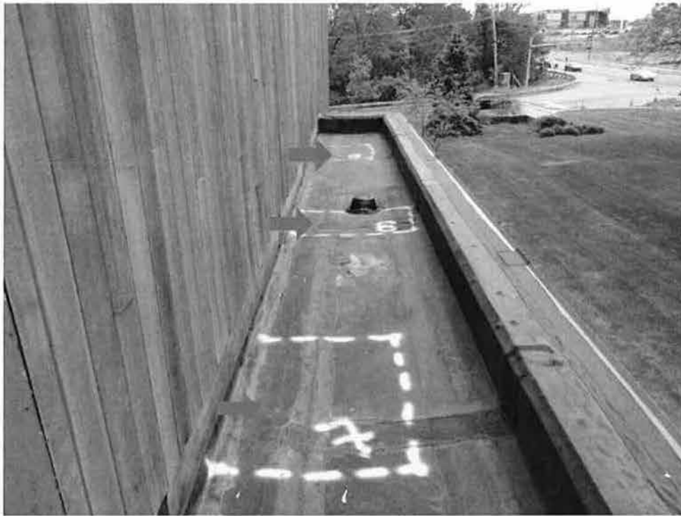
Photo 25 - Roof Area E - View of the location of water trapped in the insulated fully adhered EPDM roof system (red arrows) in Anomaly 7, 8, 9.
