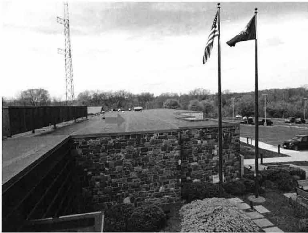
Photo 15 - Roof Area A -View of the insulated fully adhered EPDM roof system (red arrow) on Roof Area D.
