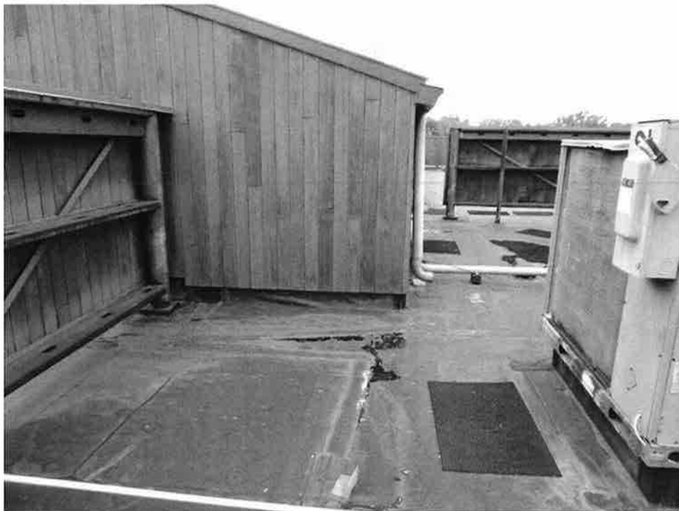
Photo 12 - Roof Area A -View of area of roof where water ponds (red arrow) on the insulated fully adhered EPDM roof system.
