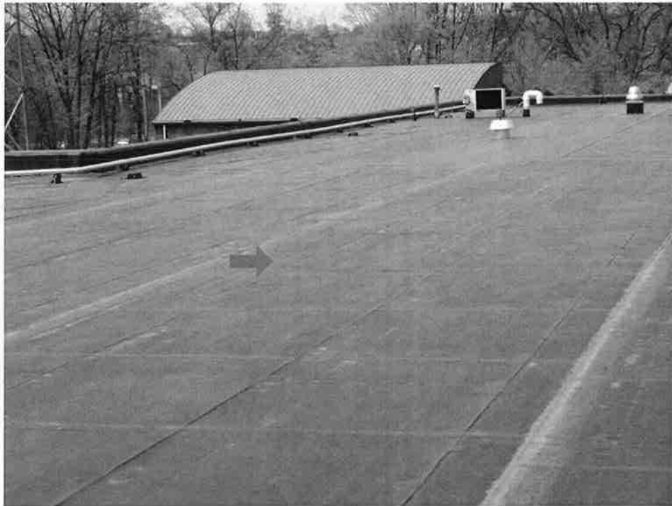
Photo 17 - View of the insulated fully adhered EPDM roof system (red arrow) on Roof Area D adjacent to Roof Area F - Canopy Roof. Nearly all of the roof surface has positive slope to the roof drains.
