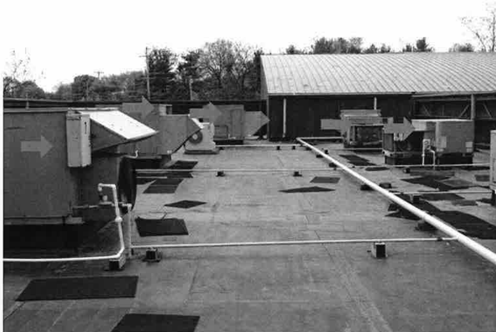
Photo 8 - Roof Area A -View of the rooftop equipment (red arrows) inside the screen wall near the roof hatch and above the insulated fully adhered EPDM roof system
