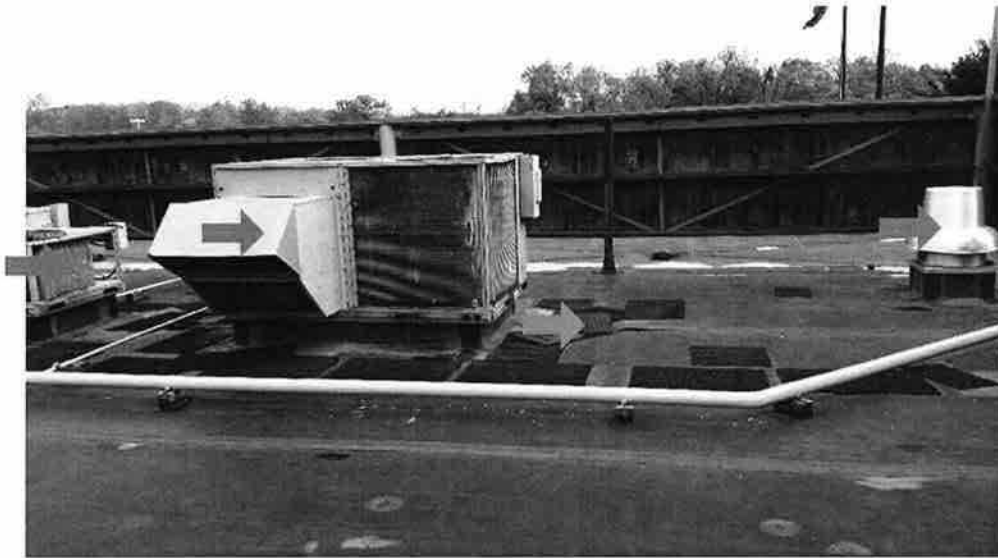
Photo 9 - Roof Area A -View of the rooftop equipment (red arrows) inside the screen wall near the roof hatch and above the insulated fully adhered EPDM roof system. Note the loose EPDM walkpads (green arrow) dispersed on the roof surface.
