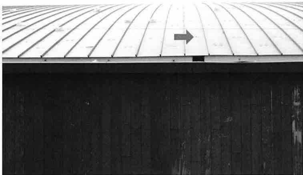
Photo 20 - Metal Roof -View of the metal roof panels where plastic snow guards have fallen from the roof (red arrow) onto the fully adhered EPDM roof below on Roof Area B.
