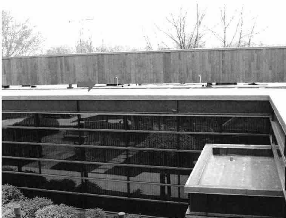
Photo 2 - Roof Area A -View of View of the insulated fully adhered EPDM roof system (refer to red arrow).
