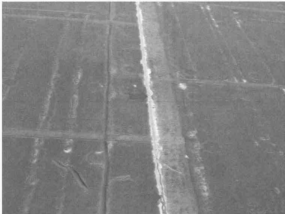
Photo 10 - Roof Area A -View of typical seam between EPDM membrane sheets (red arrows) where sealant has been installed along the edge of the seam to stop+ water leakage inside the building below.
