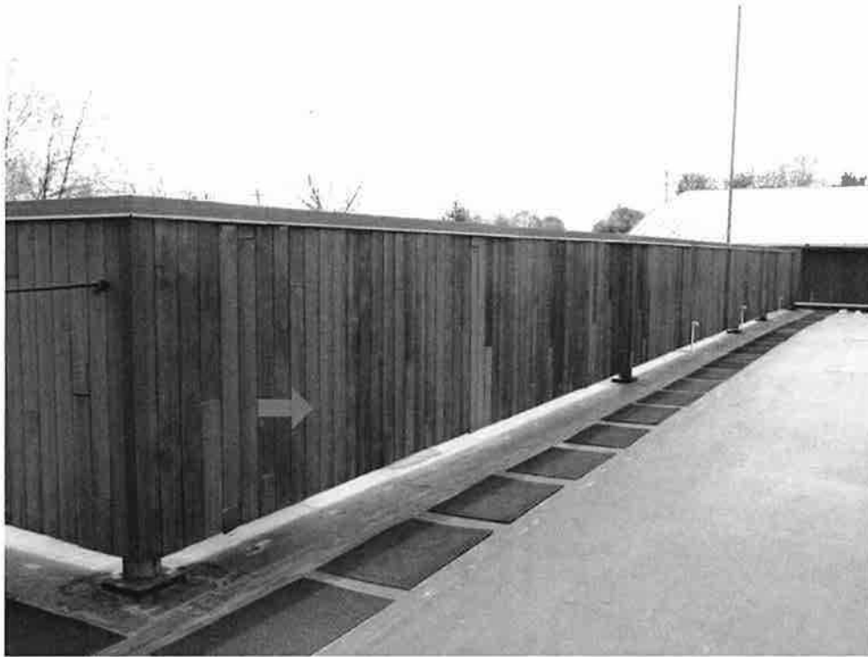
Photo 5 - Roof Area A -View of the screen wall (red arrow) above the insulated fully adhered EPDM roof system
