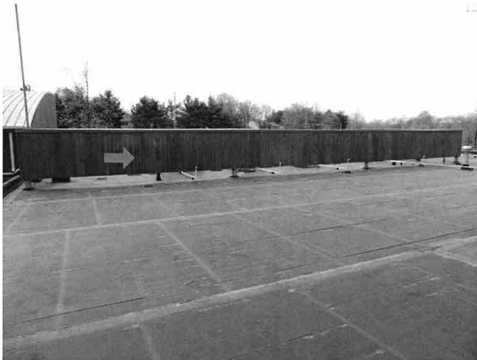
Photo 18 - Roof Area D -View of the screen wall (red arrow) above the insulated fully adhered EPDM roof system
