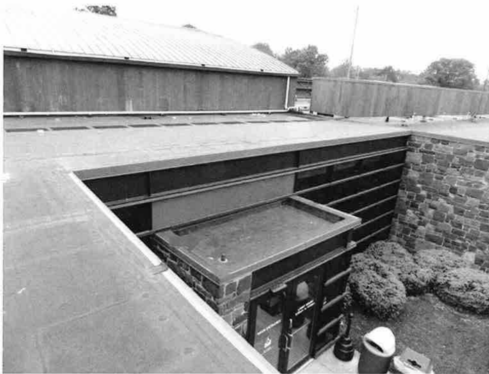
Photo 1 - Roof Area A -View of the insulated fully adhered EPDM roof system
