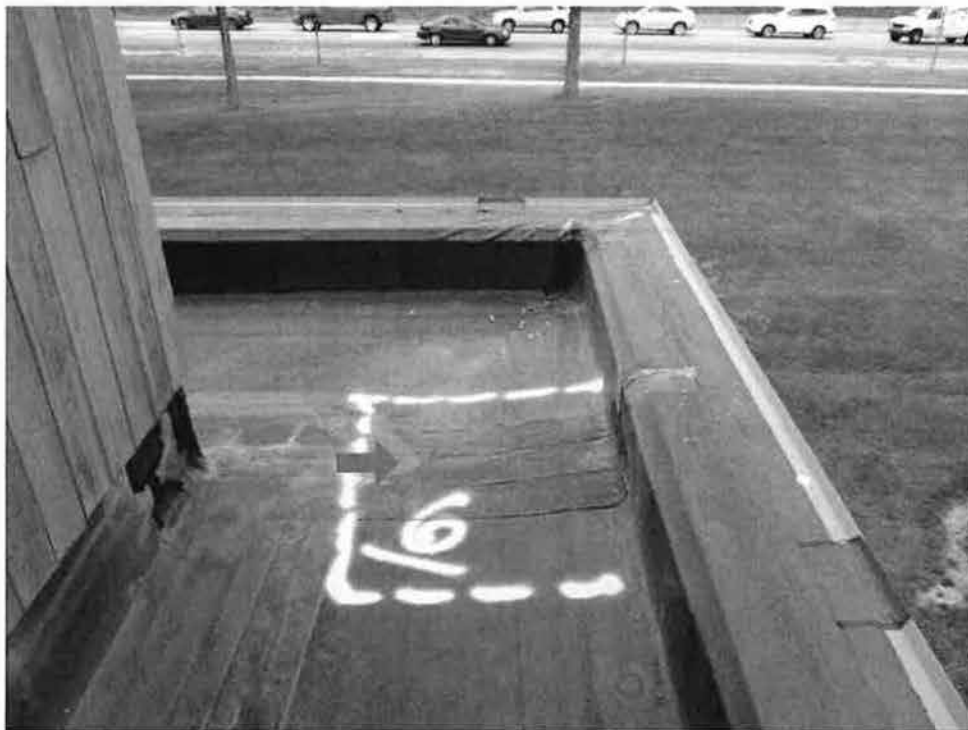
Photo 24 - Roof Area E - View of the location of water trapped in the insulated fully adhered EPDM roof system (red arrow) in Anomaly 6.
