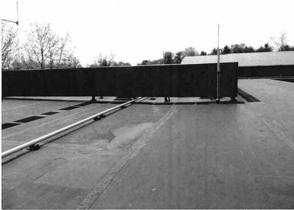
Photo 3 - Roof Area A -View of areas of roof where water ponds (red arrow) on the insulated fully adhered EPDM roof system
