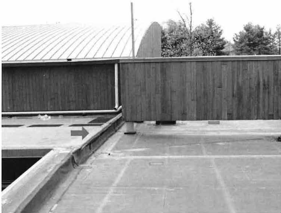
Photo 16 - Roof Area A -View of the firewall (red arrow) between sections of Roof Areas B & D.
