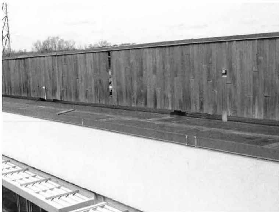
Photo 22 - Roof Area D -View of the screen wall above the insulated fully adhered EPDM roof system. Note the missing section (red arrow) of wood siding in the screen wall.
