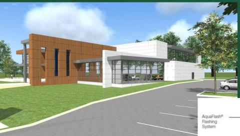
White areas on the building are proposed to be synthetic stucco otherwise known as Dryvit or EIFS (exterior insulation & finish system).
