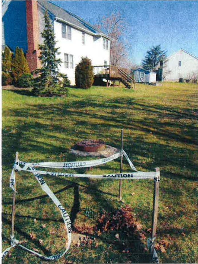
PHOTO 1 – Sink hole near storm sewer manhole up gradient from Basin No. 2.
