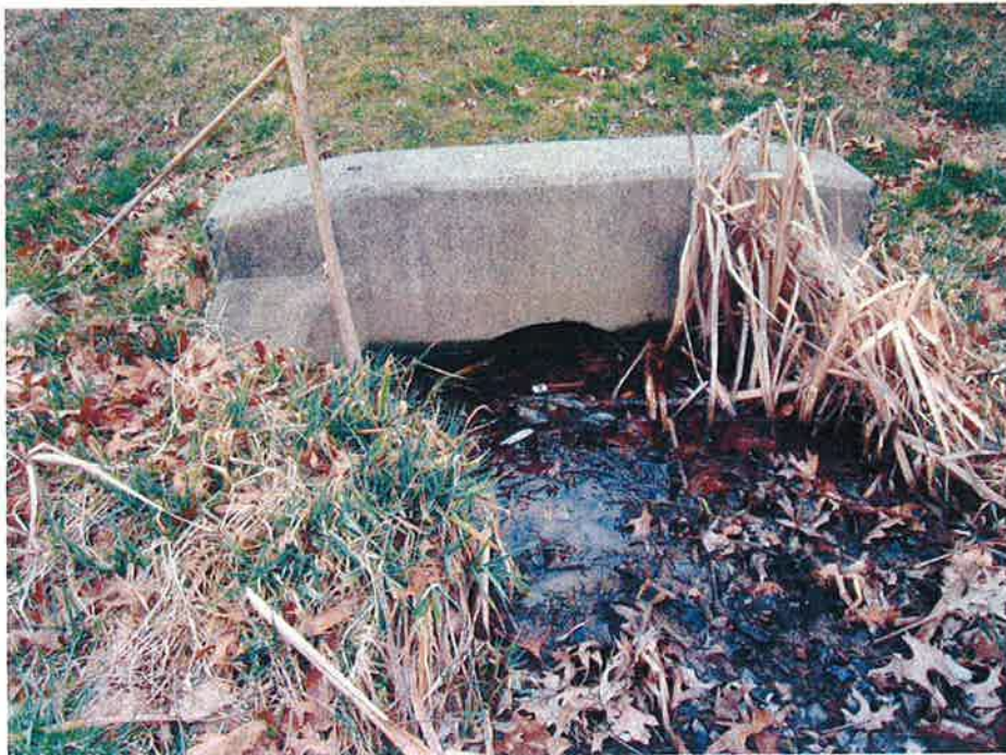
PHOTO 5 – Submerged pipe outlet.
