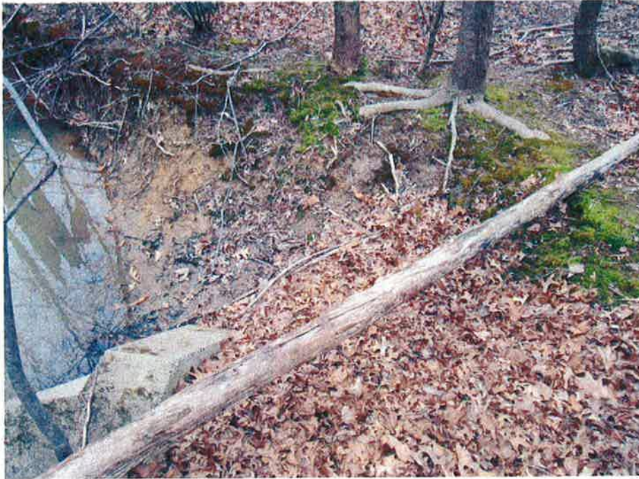
PHOTO 4 – Erosion of receiving channel.
