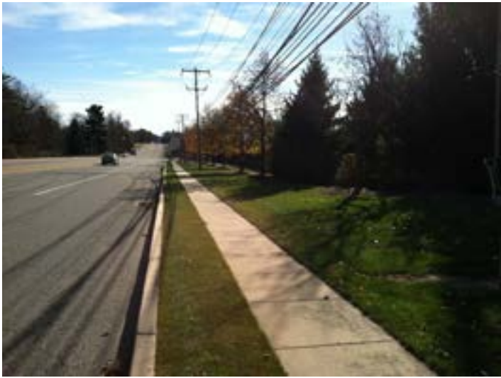
33. EXISTING WALK ALONG HORSHAM ROAD AT TEVA
