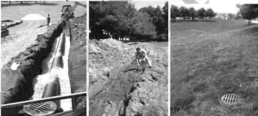
Figure 4: Example of Infiltration Trench Installation
